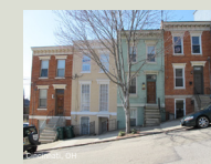
Medium-intensity character formed by a continuous street wall, vertical transparent openings, and stoops within the setback for privacy and direct street access.
