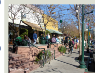
A terrace with space to sit and visit, projecting signage, awnings, entries, and transparent windows activates the public realm.
